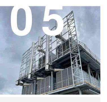
Jeremias' modular design optimised space usage, saving floor area allocated to generators and freeing up more space for the Data Hall. The complete separation of the energy building from the main server building minimised the fire protection requirements.
